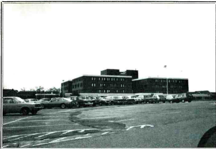
Atop this central building at a VA medical center are a number of communications antennas.
